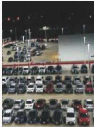
○ Parking lot Lighting
